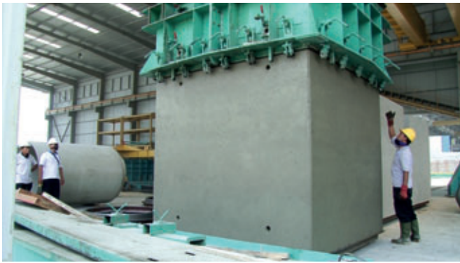
A box culvert produced on the Jumbo plant pictured during demoulding
